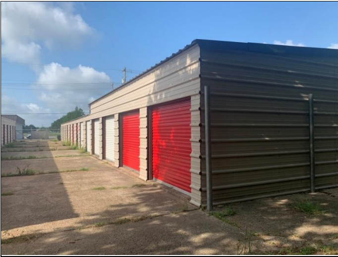
7. View of subject property building.
