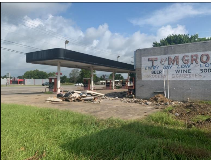
11. View of the western adjacent property.
