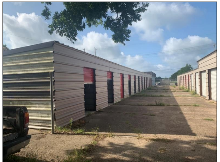
6. View of subject property building.
