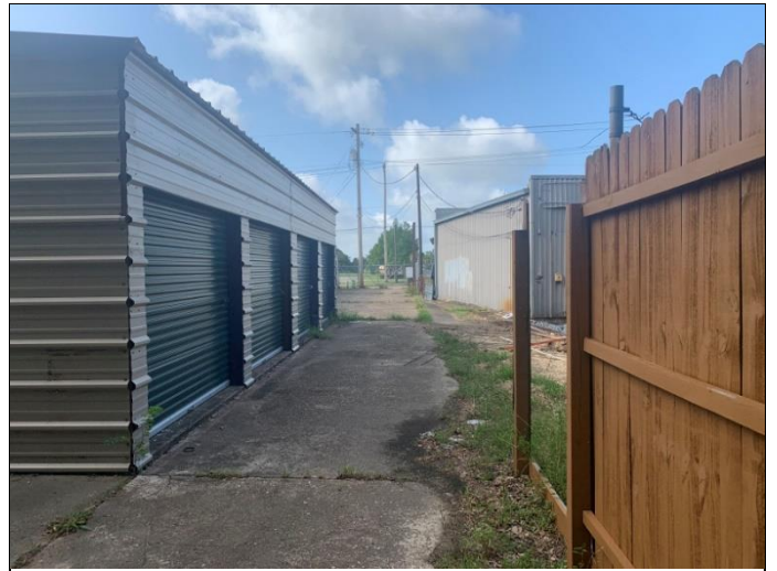
4. View of western perimeter, facing south.
